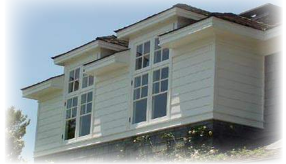
Transom windows breaking roof plane
