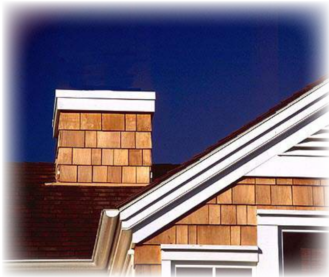
Chimneys should use materials and detailing similar to those found on building.
