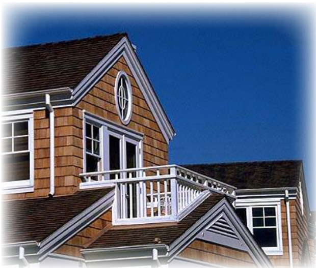
Small deck and round window help reduce mass of second story. Texture materials, siding, and divided-light windows add to composition.
