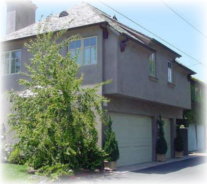
Second floor projects beyond the garage wall plane
