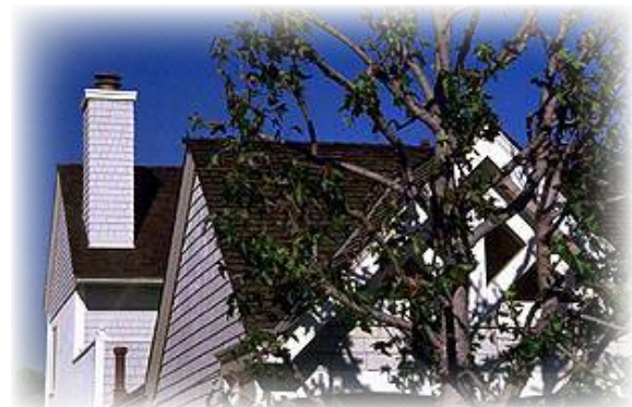
Steep roof pitches with varied heights are used on visible elevations at corners of streets.
