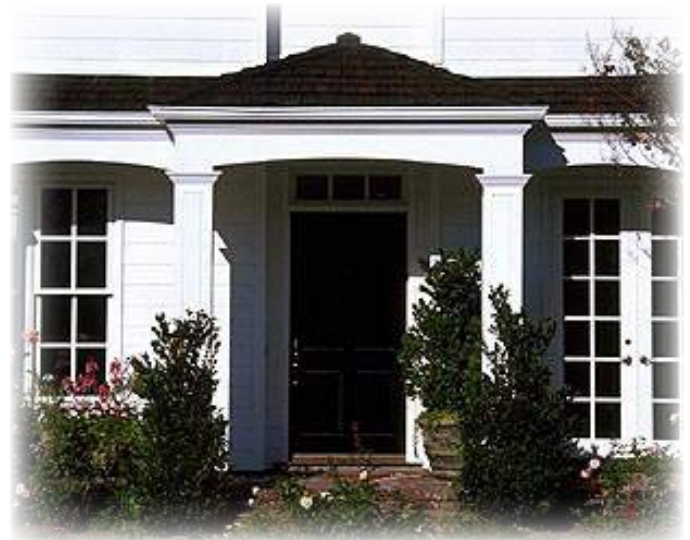
Small entry porches, columns, and low roofs are strongly encouraged to help give a sense of human scale to homes.
