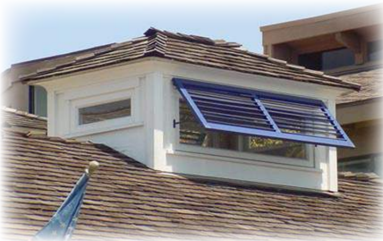
Vented roof cupola
