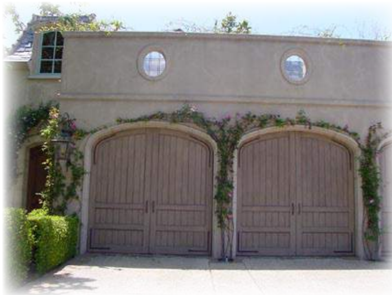
Single garage doors designed to match the architectural period
