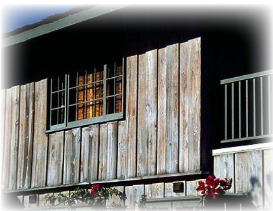
Weathered wood board and batten give a peaceful and warm feeling.
