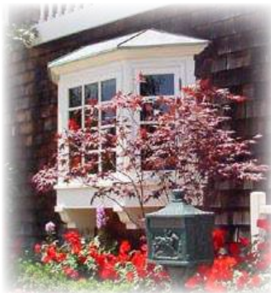
Roofed bay window
