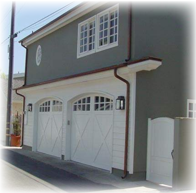
Shed roof over garage doors
