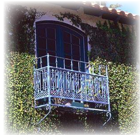
A simple attached balcony and landscape help create detail and visual interest to opening in flat wall.
