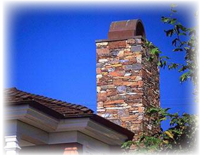
Chimney of stone and designed metal cap are used to complete the design character.
