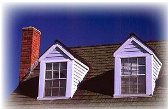
Smaller scale dormers help reduce large roof mass.
